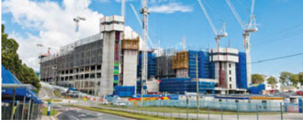
The Gold Coast University Hospital under construction
